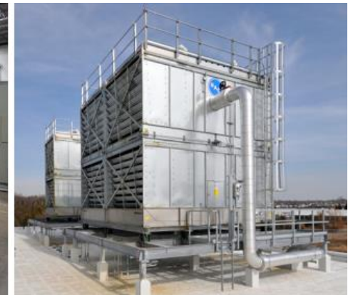
Above: Water-cooled chiller and associated rooftop cooling tower.
